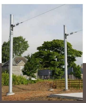
The use of trams or trolley buses is the future: it is a proven form of sustainable public transport without annoying exhaust fumes in the urban environment. Especially for this purpose we have already been able to provide many tram and trolley bus routes with poles for suspending the necessary overhead contact lines. Thanks to the overhead contact lines the passing tram or trolley bus is provided with power in a reliable manner.
